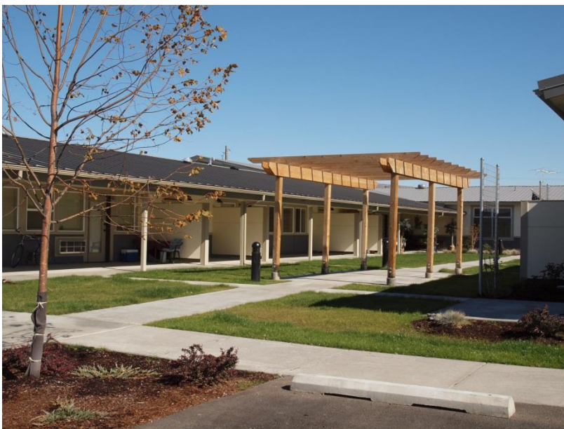
Project Name: Richmond Elementary School City: Richland Year Built: 2014 Funding Source: HOME
