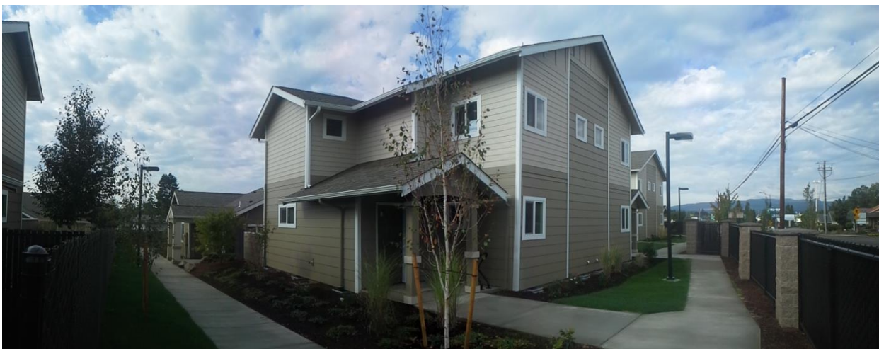
Project Name: Firestone City: Dallas Year Built: 2014 Funding Source: HOME
