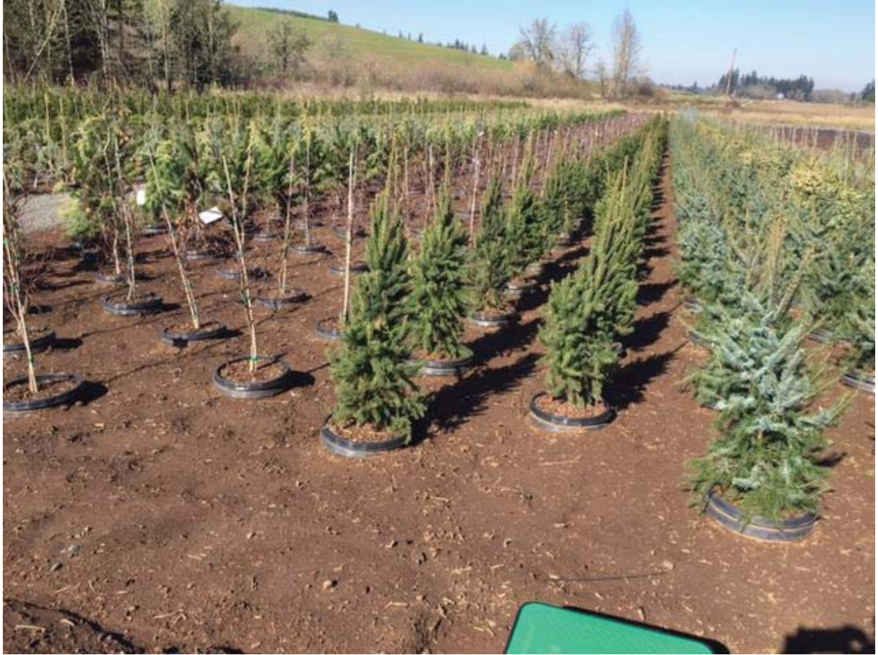
Detail with electric valve box and spray sticks.
