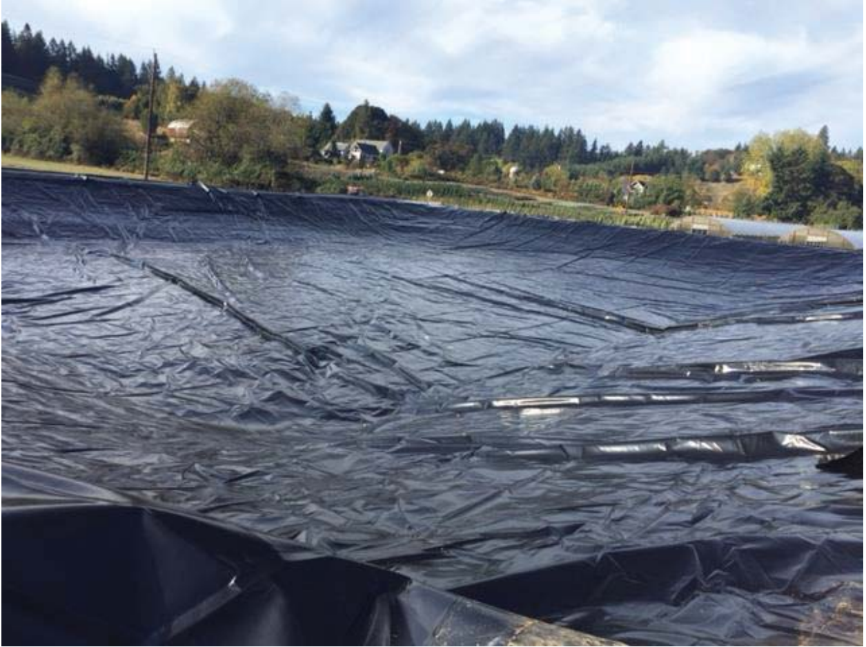
Unanticipated Liner for leaking irrigation reservoir.
