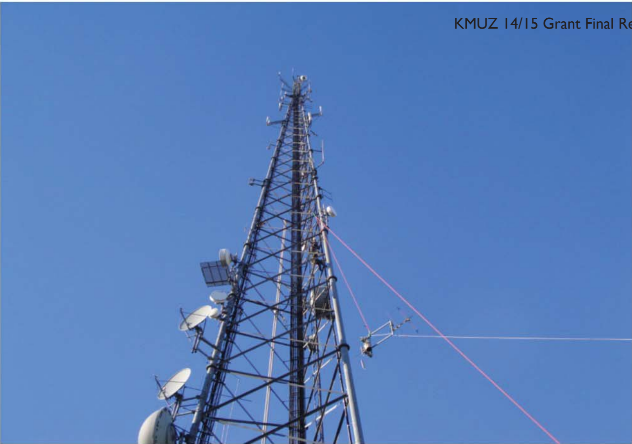
ABOVE: K264AA transmit antenna heading up to the 98' level on the Slater Sites, Inc. Prospect Hill tower.
