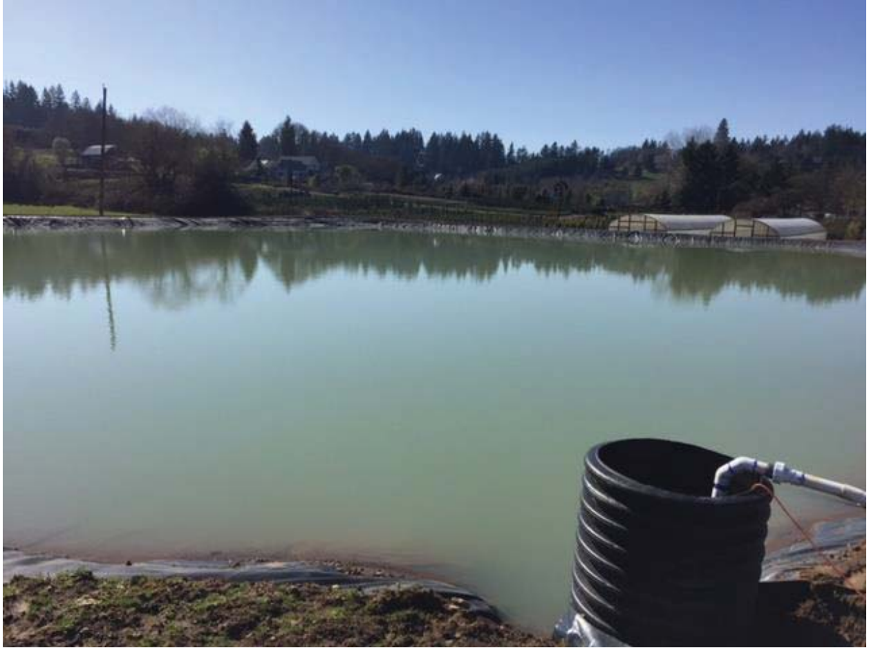
Full irrigation reservoir.
