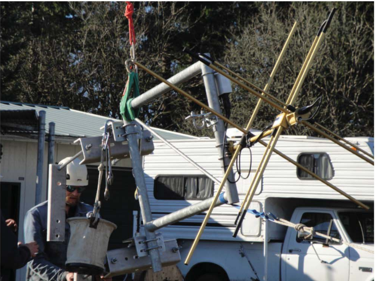
BELOW: Our Scala CA2-CP FM transmit antenna and stand off mount.
