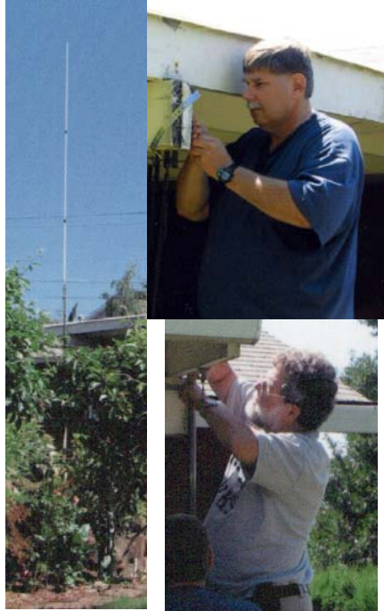
Don Busch (top) and Frank Gruber (bottom) install necessary equipment
