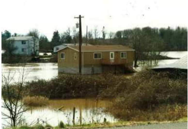
Dwelling on the Pudding River elevated to protect it from flooding.
