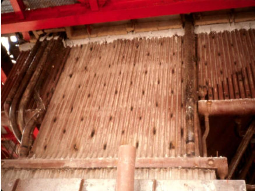
**Figure 1 - Waterwall Furnace Section<sup>4</sup>**
