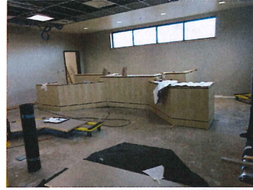
Interior progress Judge's bench with area for witness and court recorder
