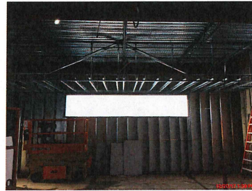
Interior progress Soffit ceiling above judge's bench
