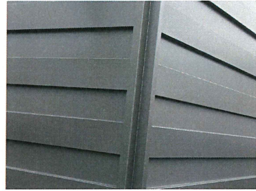
Exterior progress Trim flashing at outside corner complete
