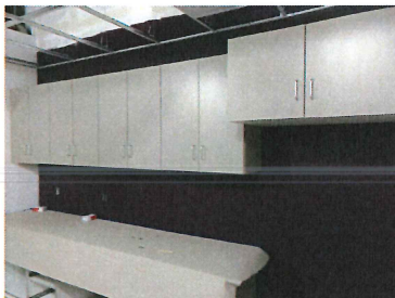
Interior progress Breakroom cabinets installed
