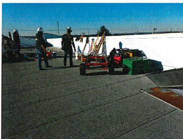
Phase 1 low slope roof Staging for stage one work
