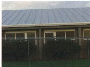
Phase 2 PVC ribs attached
