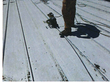
Phase 2 Machine used to cut mechanically folded metal ribs
