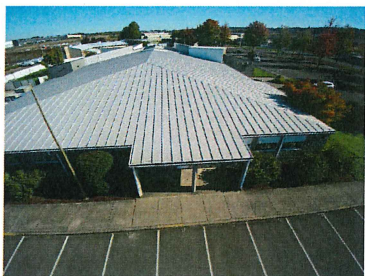
Phase 2 Drone photo of final roof
