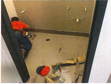
Interior progress Bathroom flooring installation
