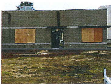
Exterior progress Glass is protected and plants have been removed
