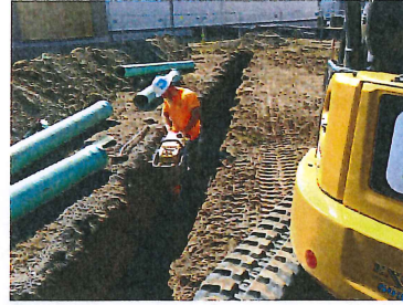
Exterior progress Storm drain piping is being installed
