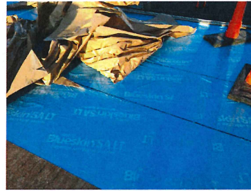
Phase 1 Self sealing vapor barrier
