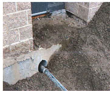
Exterior progress Final connection
