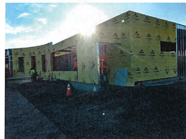
Exterior progress Structural sheathing at front hallway
