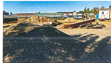
Exterior progress Excavation progress
