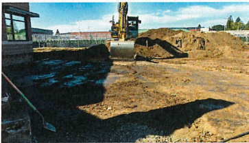
Exterior progress Cutting down to undisturbed soil for foundation pad
