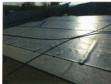
Phase 1 Roof membrane adhered before seams were welded
