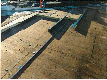
Phase 2 Old roof demo-no visible vapor barrier was present
