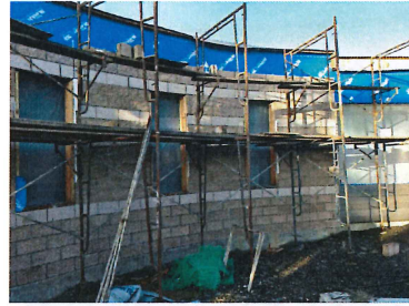
Exterior progress Continued
