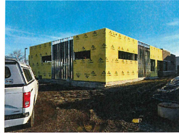
Exterior progress Structural sheathing being installed
