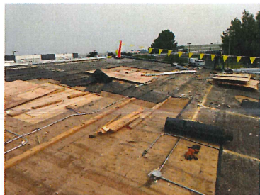
Phase 2 Demo of old shims and vapor barrier
