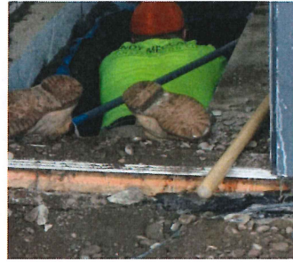
Exterior progress Getting into their work
