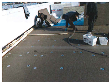
Phase 1 Placing second layer of insulation into adhesive
