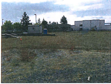
Exterior progress Construction trailer and fencing arrives on site
