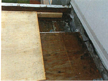
Phase 2 Spanning the soffit with plywood rather than insulation
