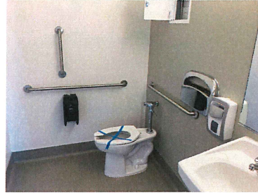
Interior progress Completed bathroom
