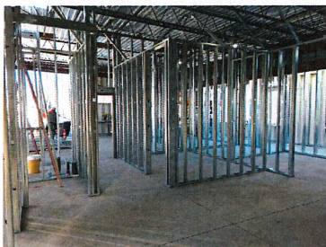
Interior progress View from old staff area toward new staff area
