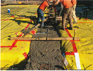
Exterior progress Pouring the spread footing
