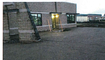
Exterior progress Final gravel for concrete pad
