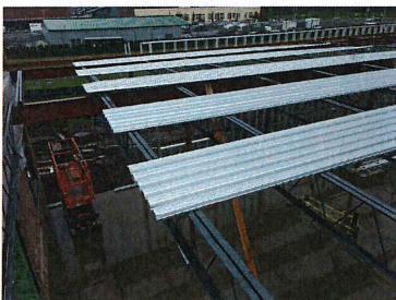
Exterior progress Installing the pan deck for the roof structure
