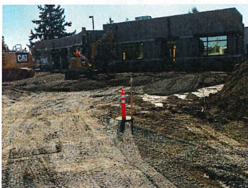
Exterior progress Placing gravel for the concrete pad
