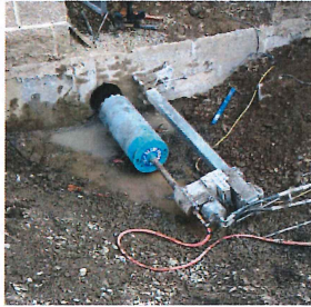
Exterior progress Drilling into old slab to access plumbing drain
