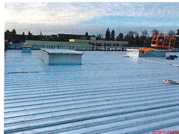
Roof progress Pan deck and mechanical curbs are completed
