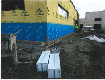
Exterior progress Starting vapor barrier and Concrete Masonry Units (CMU)
