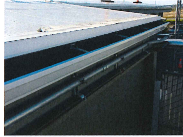
Phase 2 New gutters
