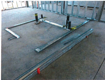
Interior progress Placing the floor track for the bathrooms
