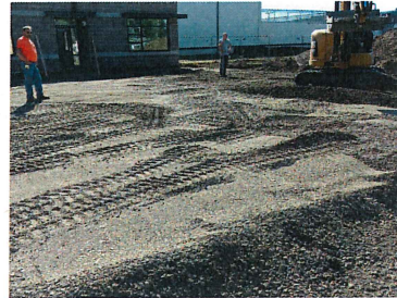
Exterior progress Final gravel placement for concrete pad
