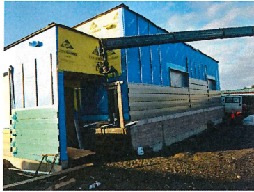
Exterior progress Installing the metal siding
