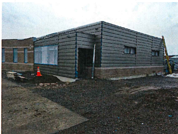
Exterior progress Siding install and trim flashing is in progress
