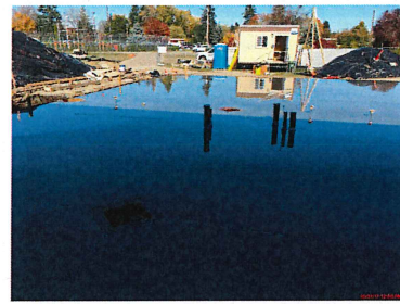
Exterior progress Water curing the slab
