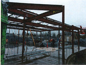
Exterior progress Raising the red iron for hallway
