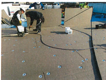
Phase 1 Adhering second layer of insulation
