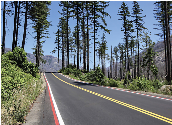
Red striping now indicates where you cannot park on or near the road shoulder.
