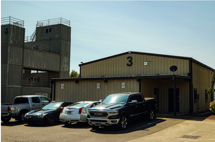
A building on the Chemeketa Brooks campus houses a well pump servicing the Brooks-Hopmere area.
