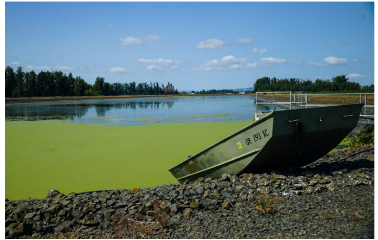
A waste water treatment lagoon located in Brooks.
