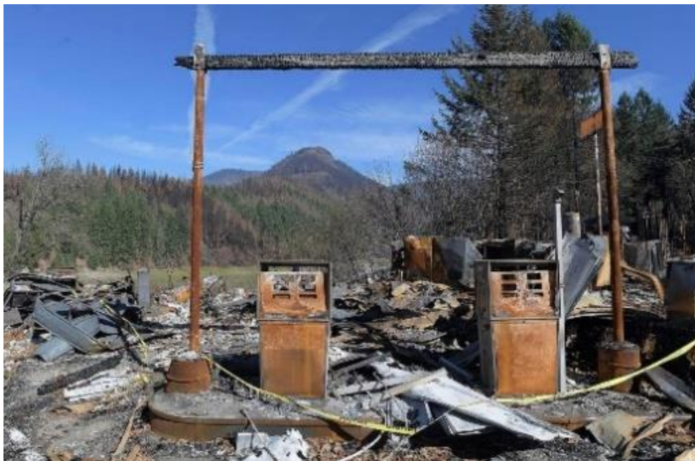
FIGURE 1-3: NORTH SANTIAM CANYON CONVENIENCE STORE DESTROYED DURING 2020 FIRES
