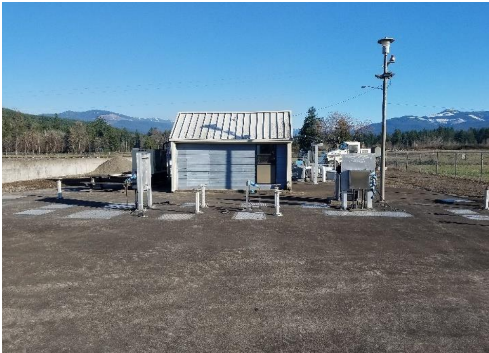
FIGURE 6-3: MILL CITY'S WATER POLLUTION CONTROL FACILITY
