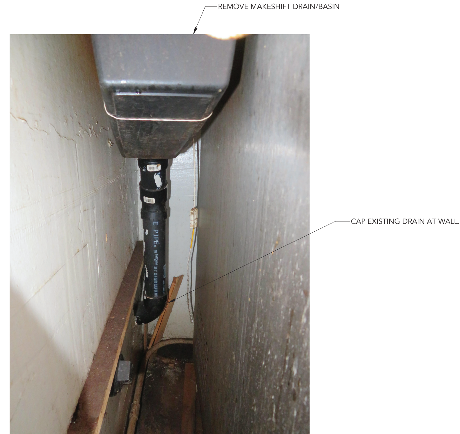
2 EXISTING ESPRESSO MACHINE DRAIN NOT TO SCALE
