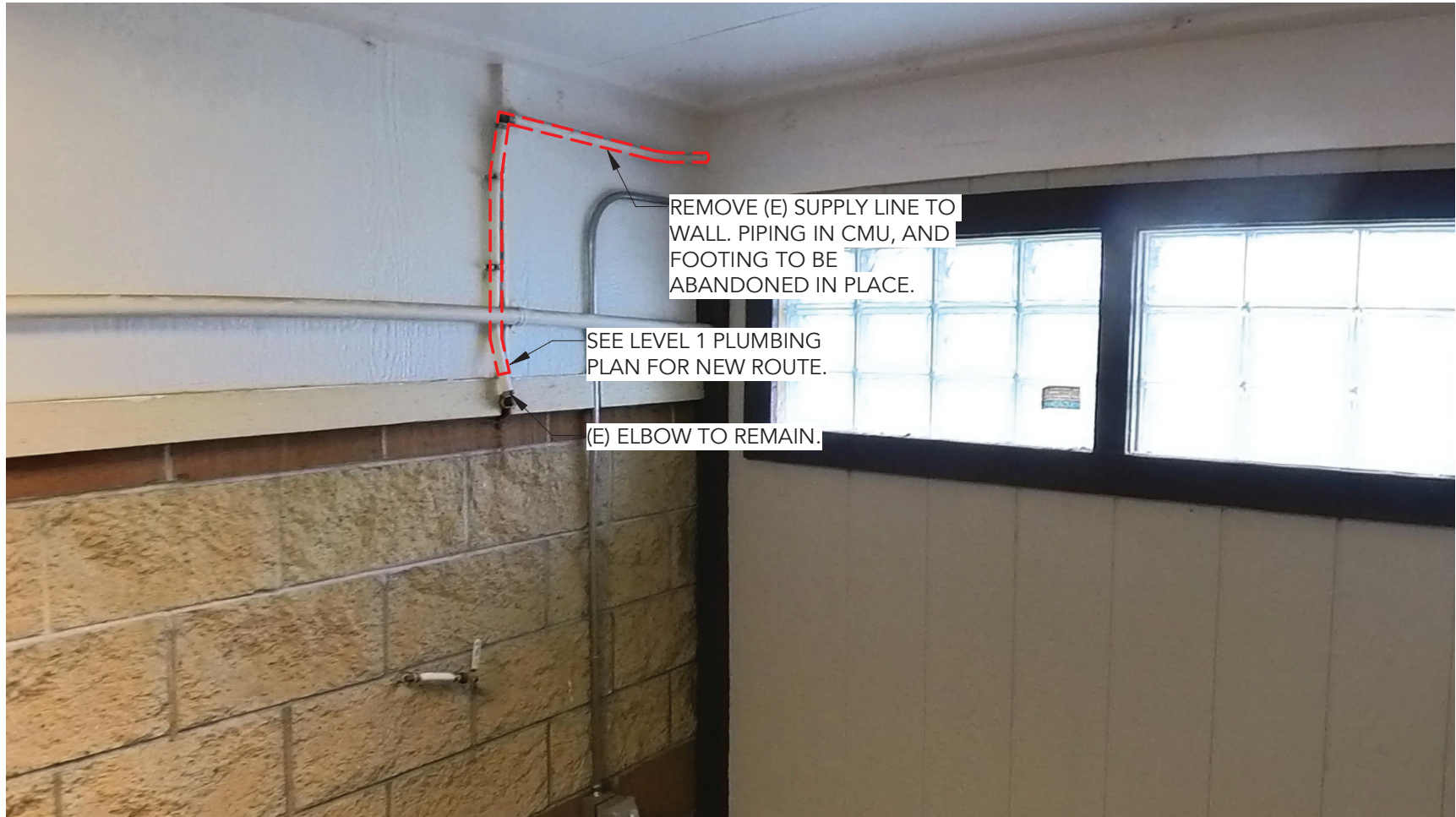
3 (E) KITCHEN APPLIANCE WATER SUPPLY REROUTE 12" = 1'-0"
