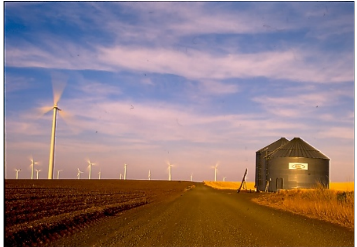
Klondike wind turbines can generate 400 megawatts of electricity
