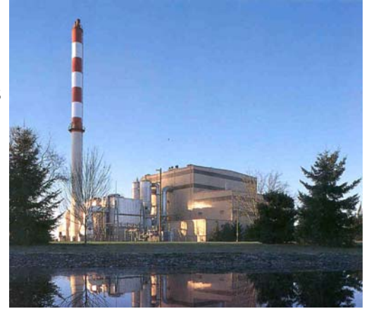
Covanta Marion's plant in Brooks, OR
