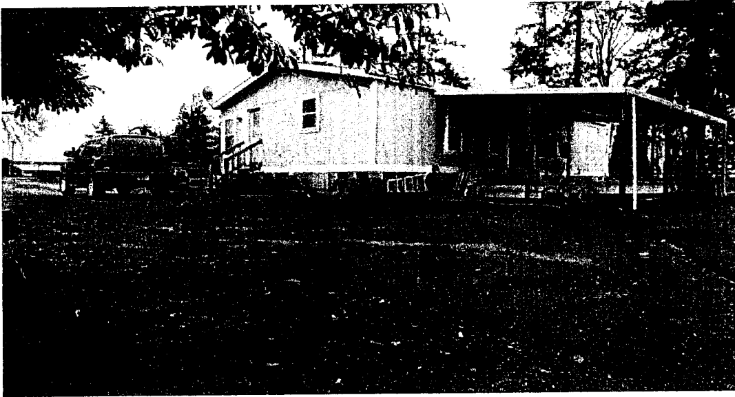
REAR VIEW LOOKING AT NORTHWEST CORNER
