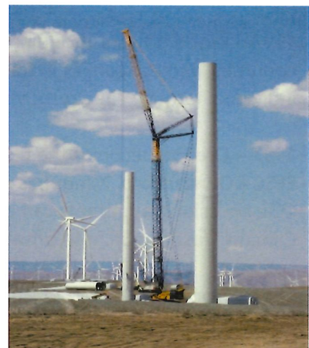
Wind turbine construction in Oregon.
