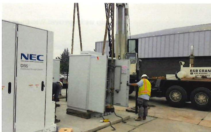
EWEB contractor installs back-up battery power system.
