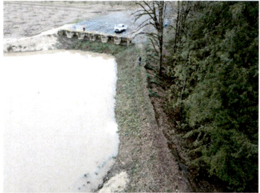
Looking south along top of berm (3/19/2025).
