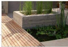
CONCRETE PLANTERS BOARD FORM SEALED CONCRETE
